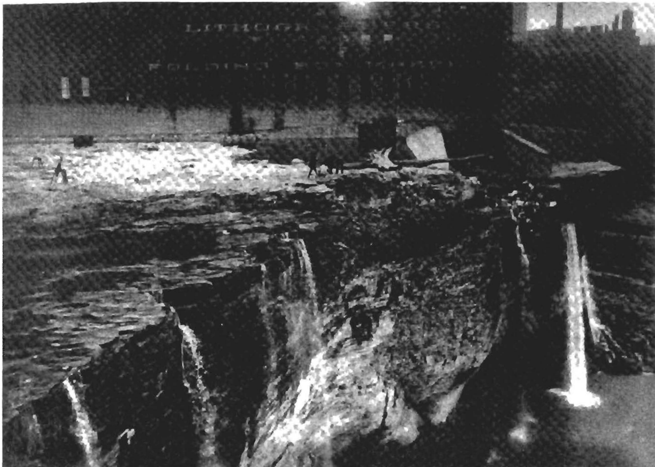
FIGURE 25 High Falls before upper ledges were removed by blasting. Looking west. Gorline Building in distance. Nov. 1914. (Stone Collection, Roch. Mus. and Sci. Center)
