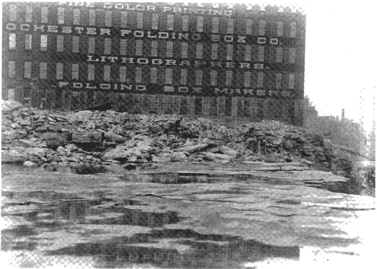
FIGURE 26 High Falls showing rock debris from blasting. Looking west. Gorsline Building in distance. Nov. 1914. (Stone Collection, Roch. Mus. and Sci. Center)
