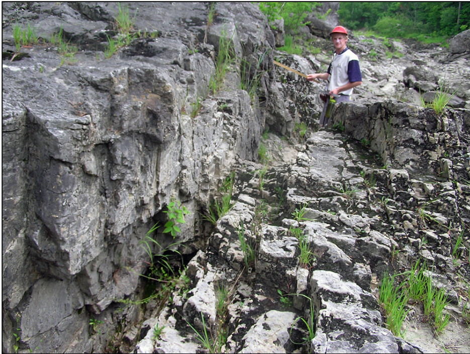
Figure 6. Northeast striking, steeply-dipping strike-slip fault zone in the Winooski River gorge.
