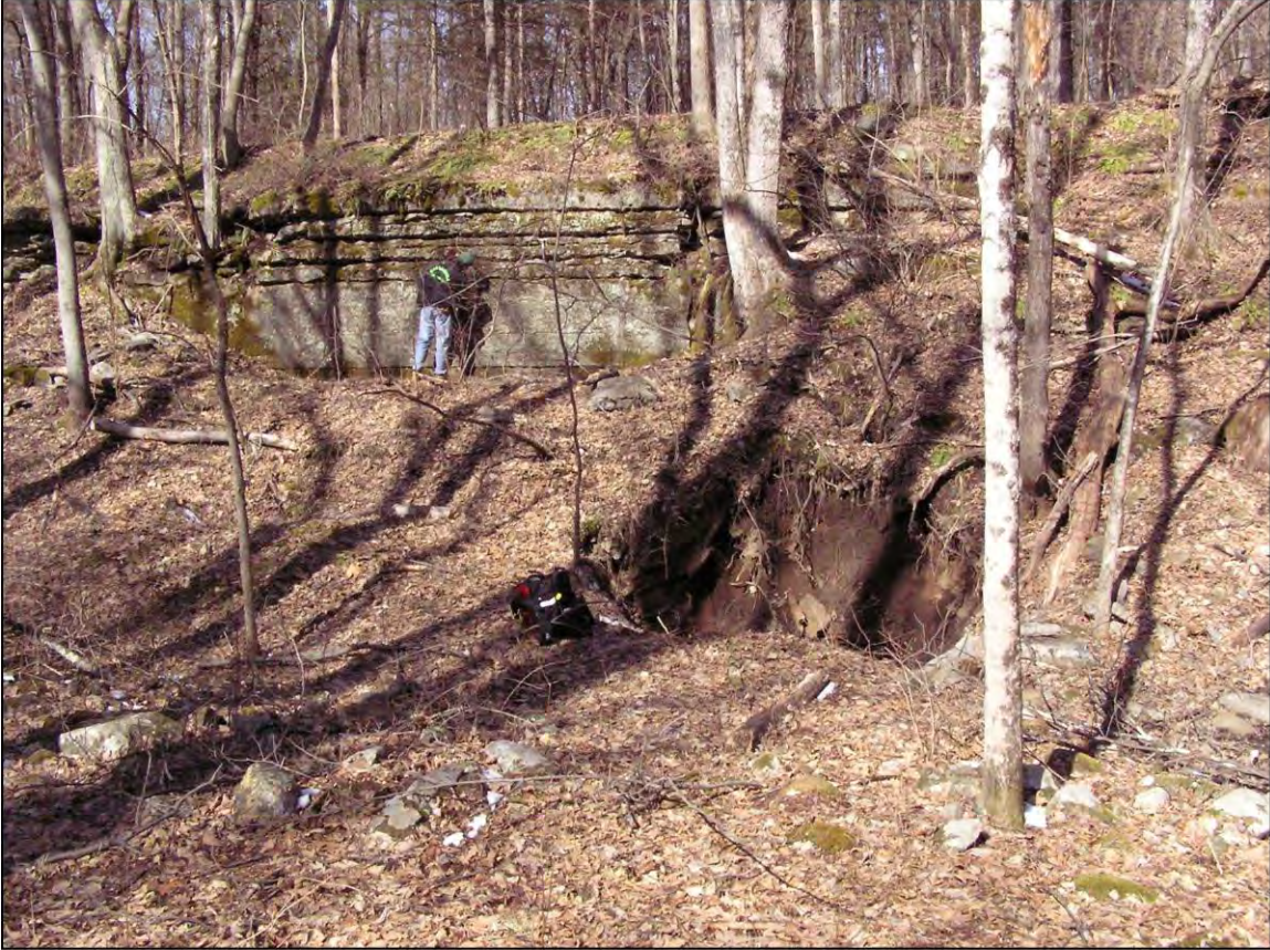
Figure 1-10. Solution collapse sinkhole over the Onondaga Limestone. Delaware Water Gap National Recreation Area. Photo by R. Witte.
