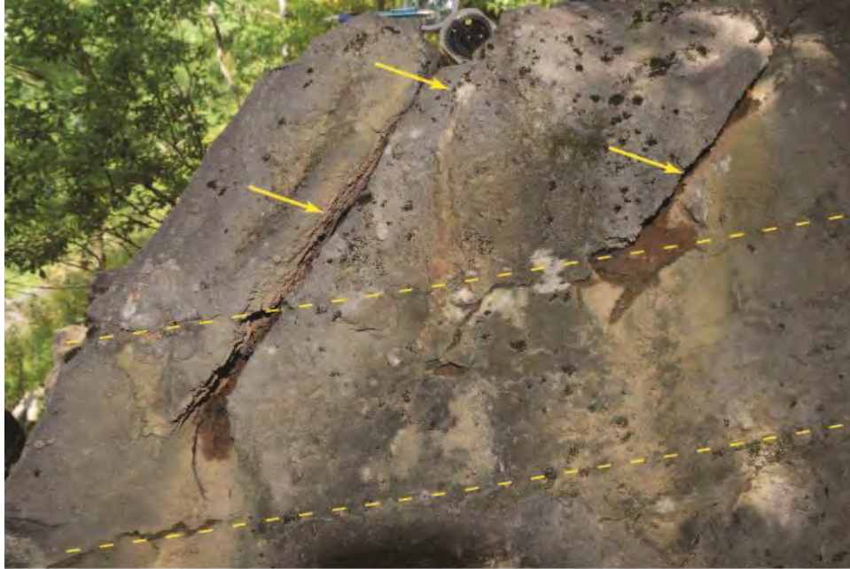
Figure 4-2. Photograph looking north at a cross joint surface within the Coeymans Fm limestone that exposes two different solution gaps identified by arrows created by dissolution of calcite-filled discontinuous veins. Third arrow locates a calcite vein that slowly dissolving. Dashed line identify bedding trend. Pencil and geologic compass for scale.
