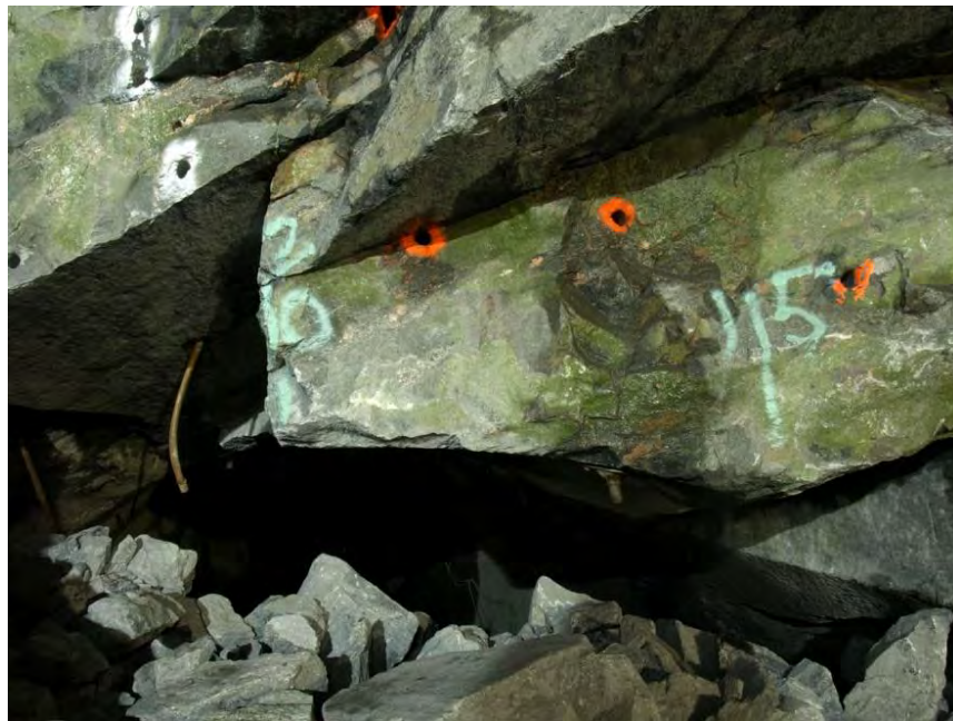
Figure 15 - View of microcrystalline epidote (green) and overgrown K-feldspar mineral coating on NW-trending joints cutting Hartland rocks above southbound TBM tunnel. (Digital image taken 19 December 2012.)
