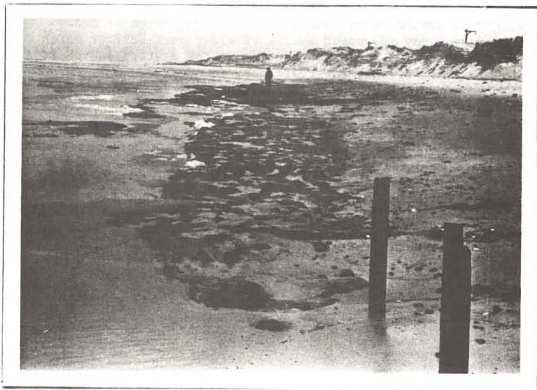
Figure 3B. Eroded beach foreshore exposing remnant pilings of Gilgo Beach Pavillion and salt marsh layer (April, 1973).
