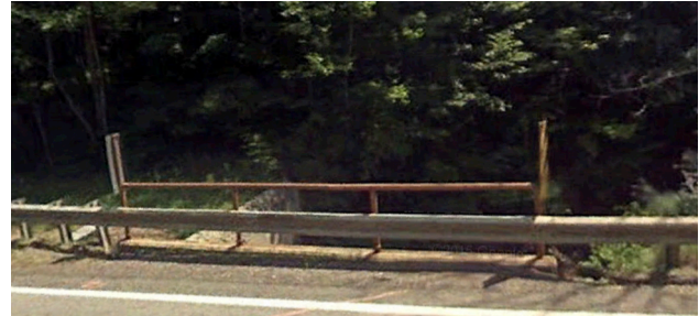
Figure 19. Bridge in 2009, before being rebuilt.
