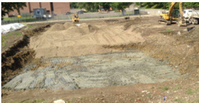
Figure 16. The clay layer extends from the Creek beneath the entire Ceramics Museum. Toward the right you can see it beneath the fill they put above.
