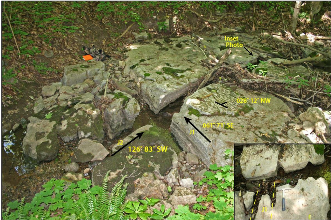
Figure 1-16. Solution joints in the Onondaga Limestone's Edgecliff Member just upstream from a small swallow hole and downstream from culvert 1. Water flows from left to right, rock hammer and fieldbook for scale. Inset photo shows dentate solution weathering along J1 joints. Water flow is right to left with hammer for scale. Photos by R. Witte.
